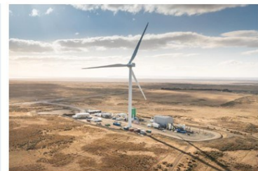
Haru Oni Pilot Plant - Punta Arenas, Chile
